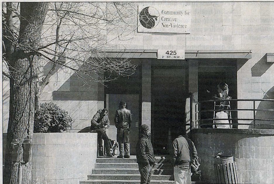
Renovations prevent CCNV from taking in new residents at this shelter on 2nd and D streets, NW.
